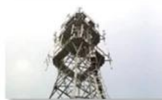
Mobile plant maintenance
