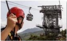
Cable car maintenance
