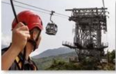
Cable car maintenance
