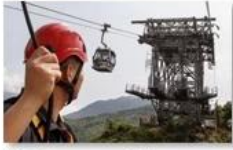
Cable car maintenance
