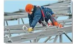
Work at height
