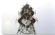
Mobile plant maintenance
