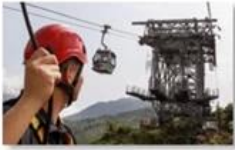
Cable car maintenance
