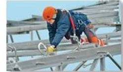
Work at height
