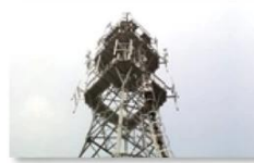
Mobile plant maintenance
