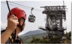
Cable car maintenance
