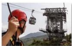
Cable car maintenance
