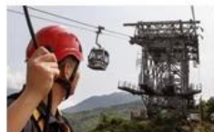
Cable car maintenance
