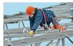
Work at height
