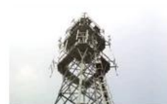
Mobile plant maintenance
