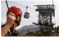
Cable car maintenance
