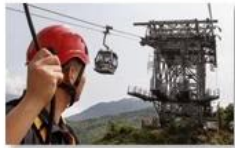
Cable car maintenance
