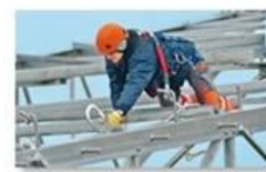
Work at height
