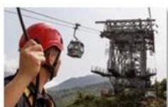
Cable car maintenance
