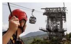
Cable car maintenance
