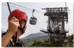
Cable car maintenance
