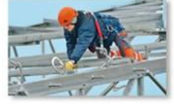
Work at height
