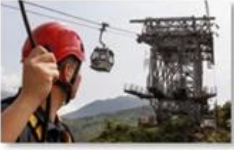
Cable car maintenance
