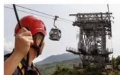
Cable car maintenance
