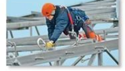
Work at height
