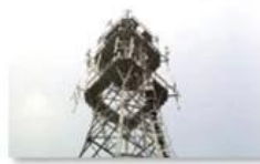
Mobile plant maintenance
