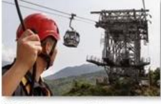
Cable car maintenance
