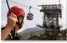
Cable car maintenance
