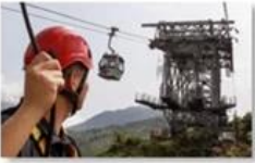
Cable car maintenance
