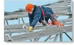
Work at height
