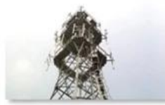
Mobile plant maintenance
