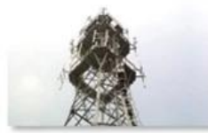
Mobile plant maintenance
